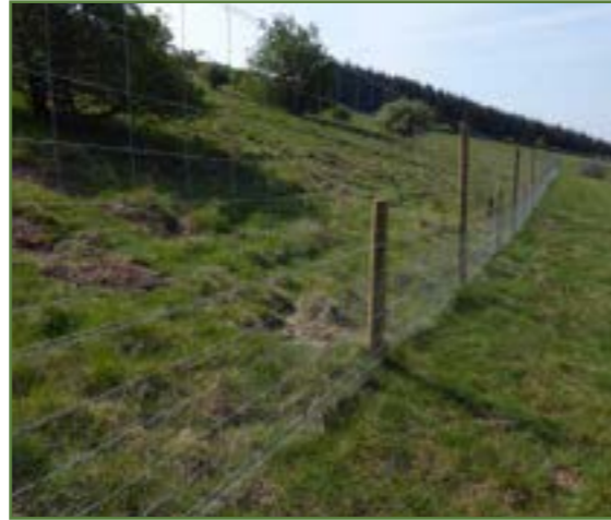
Recently installed Deer fencing
